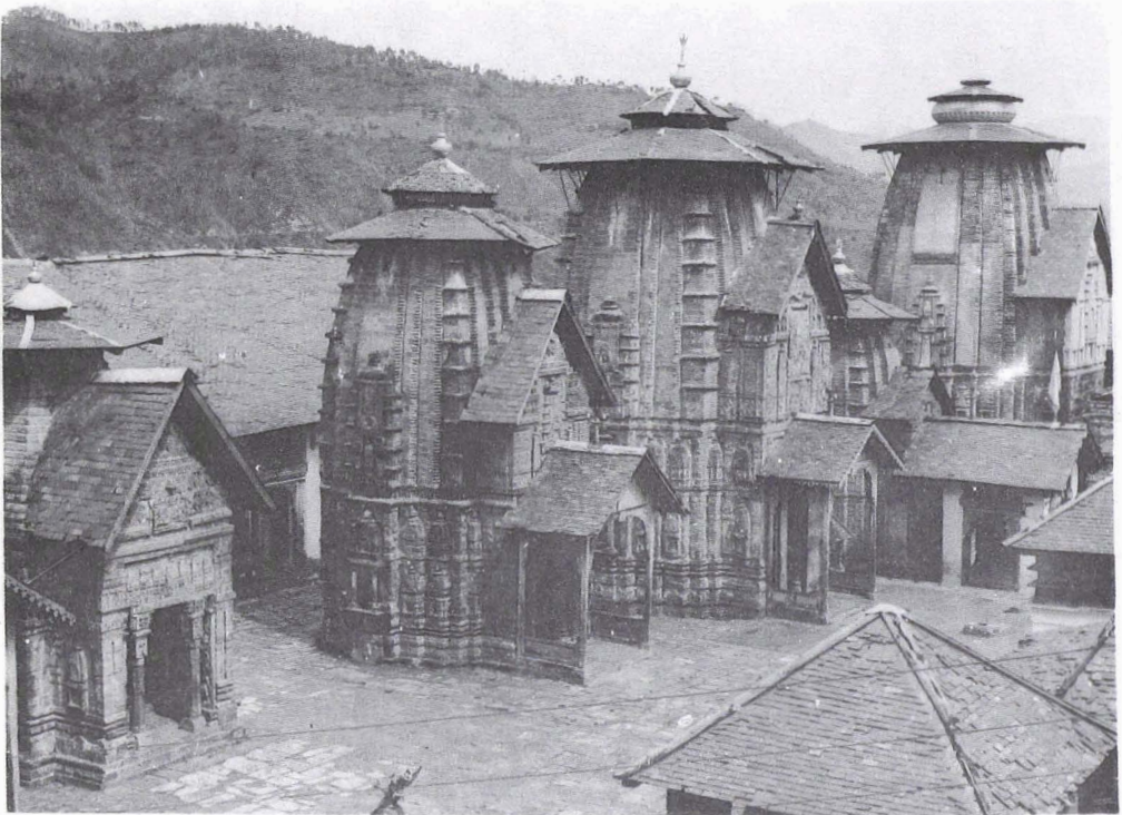
PLATE 3—Five Śikhara temples with Chatra attachments of wood and slate that were first employed in the 17th century are found in the central temple square of Chamba town. The temple of Gaurī-Saṅkara is second from the left and the temple of Lakṣmī-Narayanā is on the far right. (Copyright Archaeological Survey of India)
