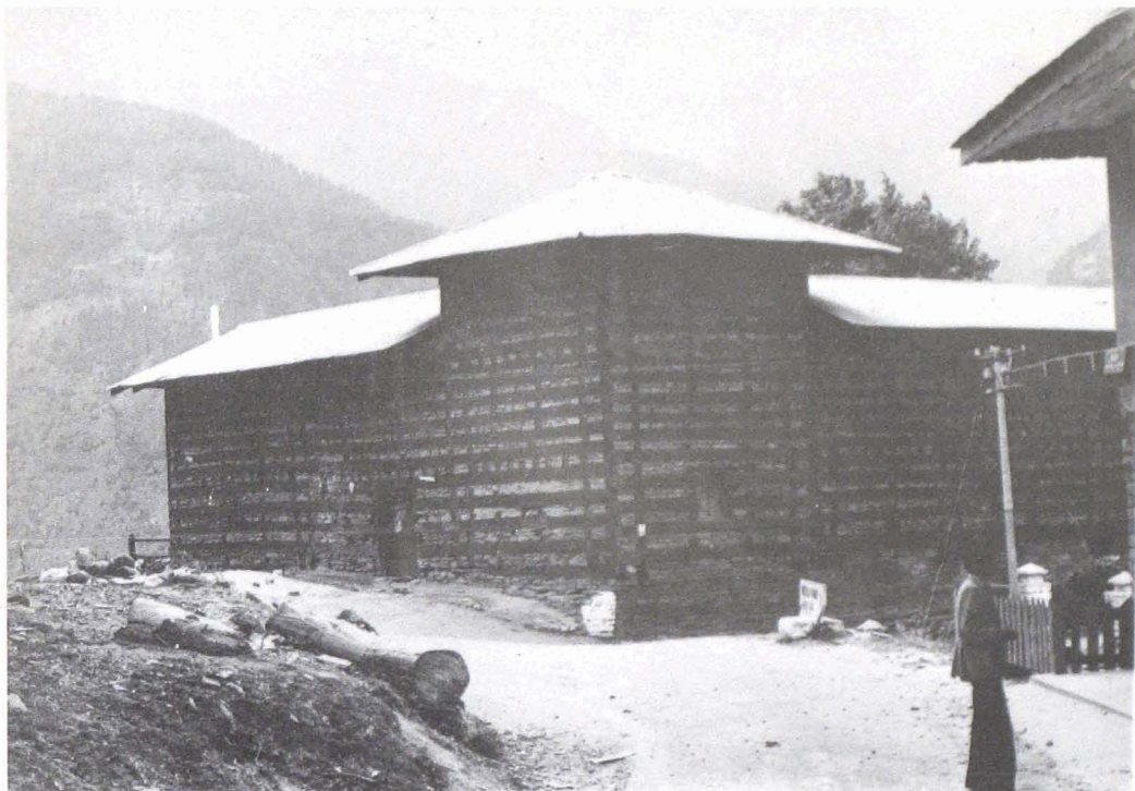
PLATE 7— Timber-bonded castle at Naggar above Kulu Valley, a massive compound that J.C. French believed to be haunted.
